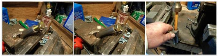
Once the bushing pops out about halfway, you can use softer blows to finish removing the bushing (and not drop and ruin the bolt threads). <sup>13)</sup>
